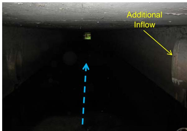
b. Box culvert which conveys channel beneath US 19
